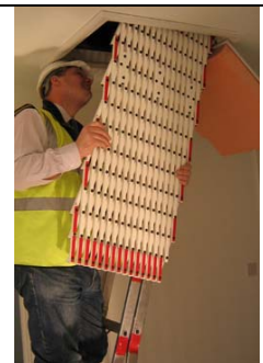
Inserting closed mat through roof space hatch
