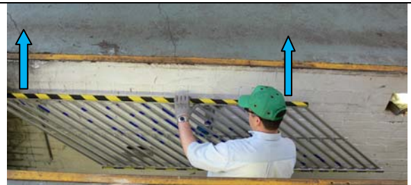
Point 14. Raising lattice upwards
