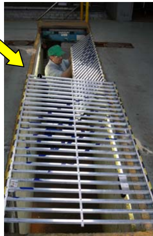
Point 6. Corner raised
