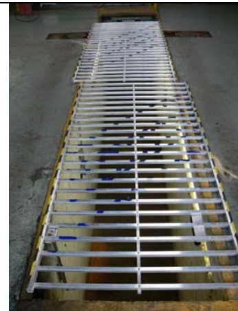
Point 2. Make a visual check of covers
