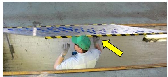
Point 15. Hinging lattice into horizontal plane
