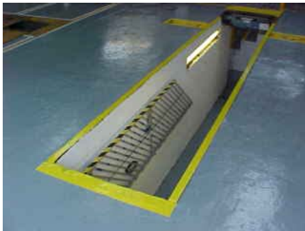
CAVE covers are retracted onto the side walls of pit – leaving full space for work
