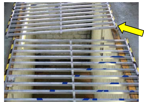
Point 5. Raise a corner
